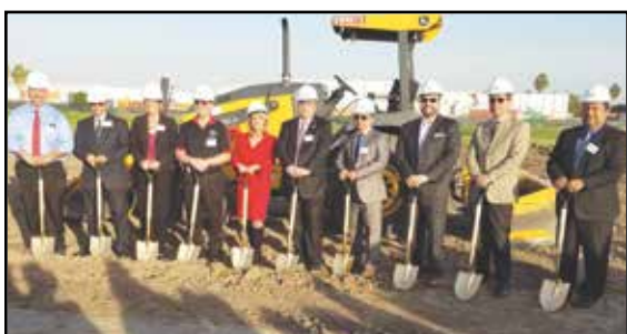
Helping break the ground for the new athletic area at John Glenn High School were members of the NLMUSD School Board, Norwalk Vice Mayor Leonard Shryock and NLMUSD Superintendent Dr. Hasmik Danielian.
