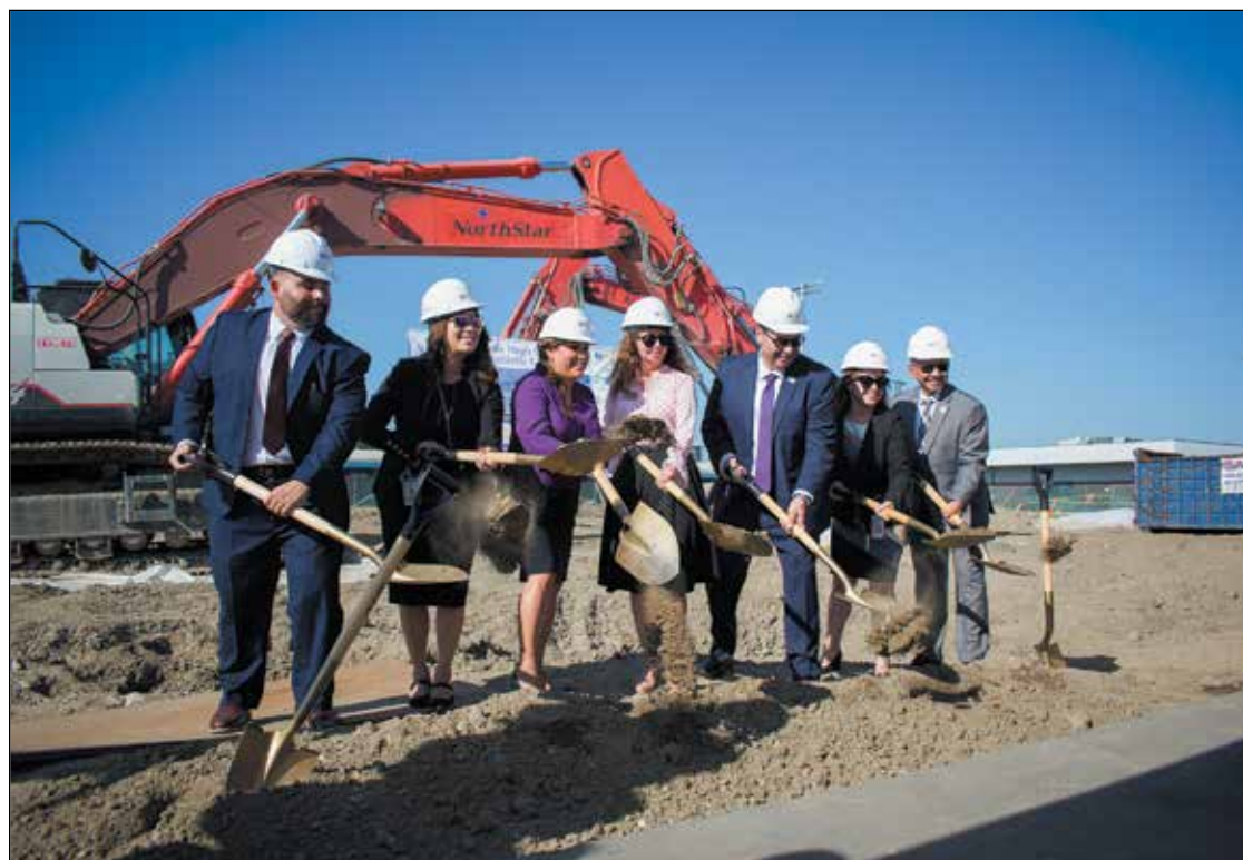
Members from the NLMUSD board of education and Norwalk High faculty break ground on a new athletic facility on Wednesday. (PHOTO BY VINCENT MEDINA)
