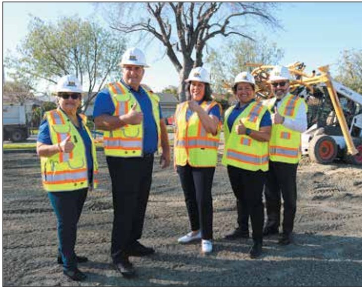
Superintendent Dr. Crean, Board President Manuel Cantu, Board Vice President Gina Ramirez, Board Members Hilda Zamora, and Jasmine Sanchez at playground construction site.
